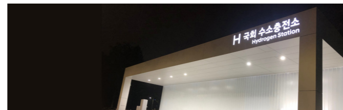
Hydrogen charging station at the National Assembly
