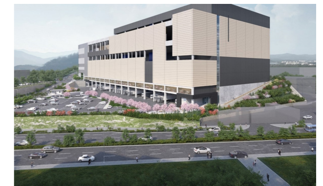
Dongtan warehouse center bird's-eye view
