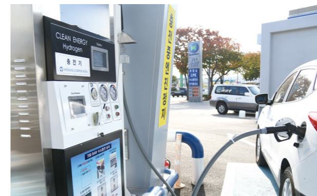
Hydrogen charging station by Hyosung Heavy Industries
